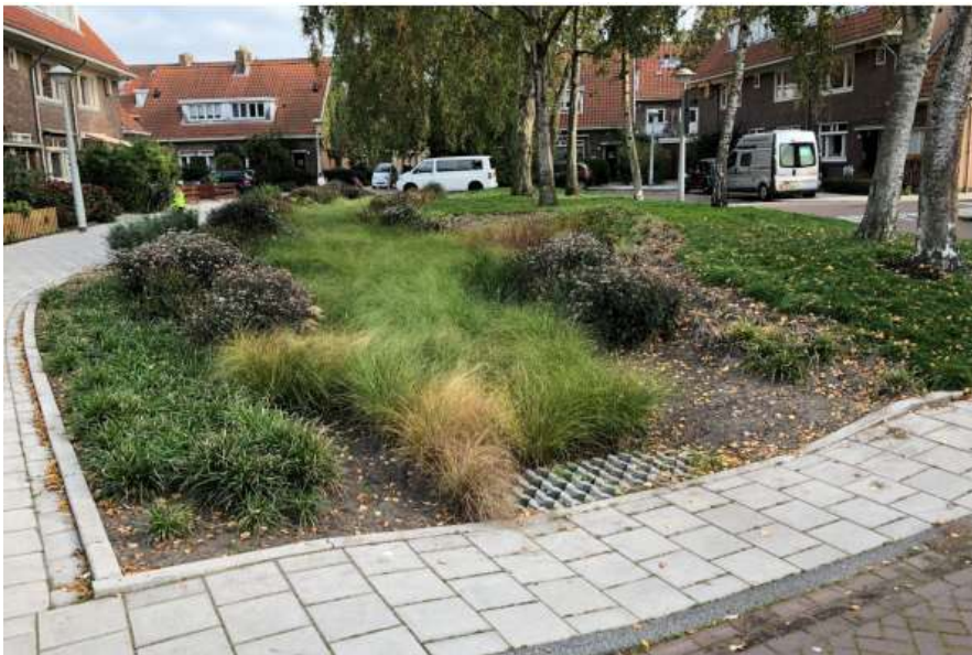
Raingarden – may be a Step 1 (single lot measure) and/or a Step 2 (urban district measure)
