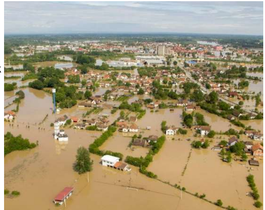
Photo: Southwestern Romania was hit by severe flooding in June 2014
